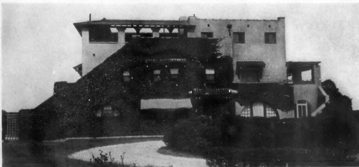
HOUSES AT "BAYBERRY POINT," ISLIP, L. I., N. Y. ESTATE OF H. O. HAVEMEYER, ESQ.
