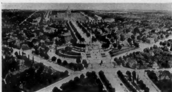
Soldiers' Monument Site, Minneapolis, Minn. Mr. Cass Gilbert, Architect.
