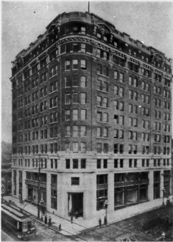
White Building, Seattle, Washington. Howells & Stokes Architects
