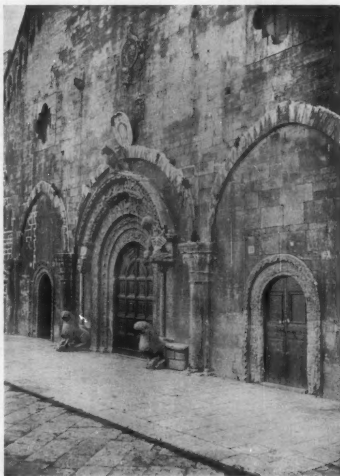
DETAIL OF THE CATHEDRAL AT RUVO
