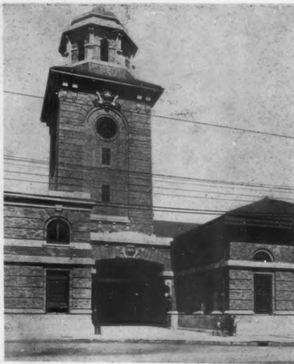
DETAIL OF NORTH TOWER
