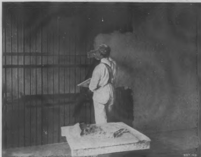
Plastering Lath Surface of HY-RIB
