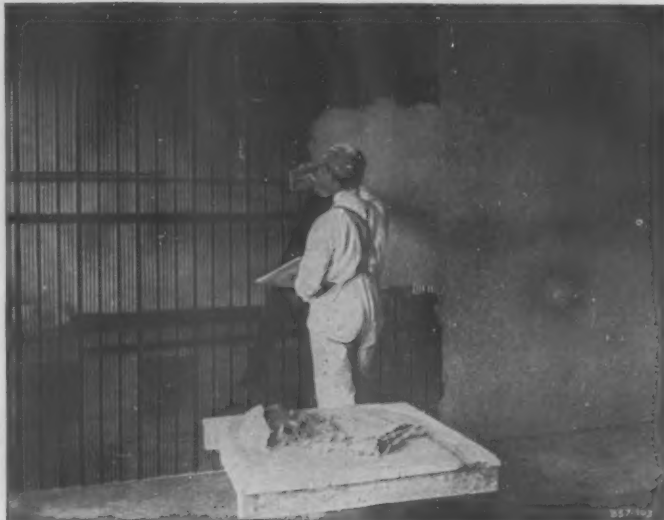
Plastering Lath Surface of HY-RIB
