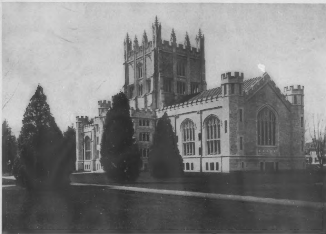
Allen & Collens Architects Boston
