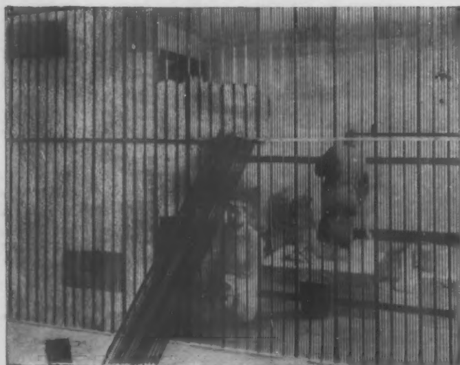
Reverse Side, Showing Perfect Key for Plastering No Dropping of Plaster
