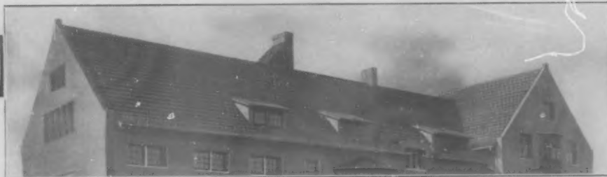
Asbestos "Century" Shingle Roof—Private Stable, Pabst Farms, Oconomowoc, Wis.; Fernekas & Cramer, Milwaukee, Architects; Constructive Sheet Metal Works, Milwaukee, Roofing Contractors
