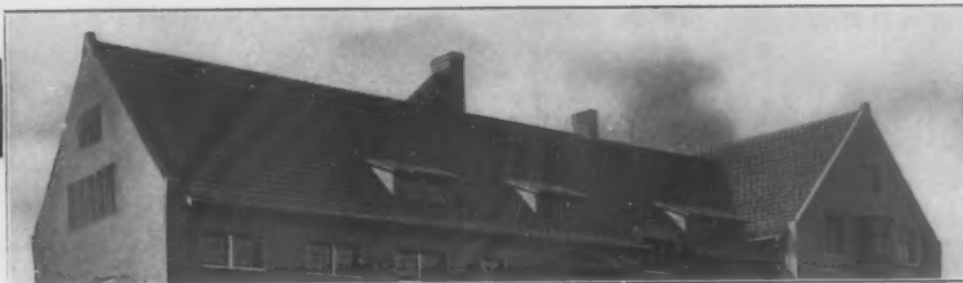
Asbestos "Century" Shingle Roof—Private Stable, Pabst Farms, Oconomowoc, Wis.: Fernekas & Cramer, Milwaukee, Architects; Constructive Sheet Metal Works, Milwaukee, Roofing Contractors
