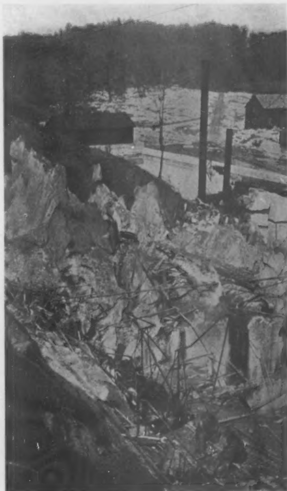
CREOLE QUARRY NO. 4 OF GEORGIA MARBLE CO.
