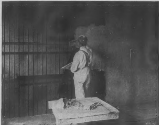
Plastering Lath Surface of HY-RIB
