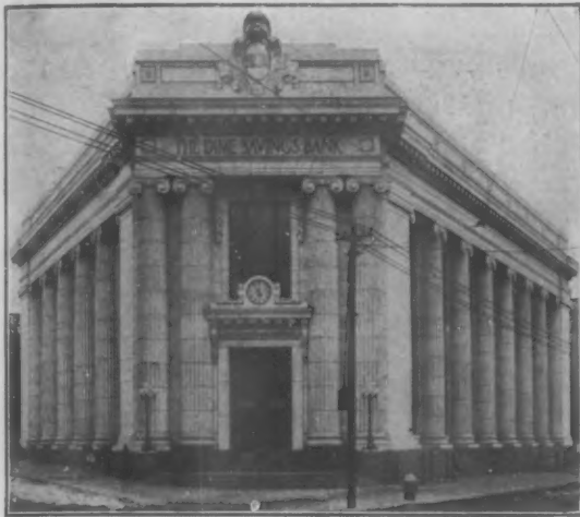
The Dime Savings Bank, Brooklyn, N. Y. Berger's Sidewalk Lights Installed
