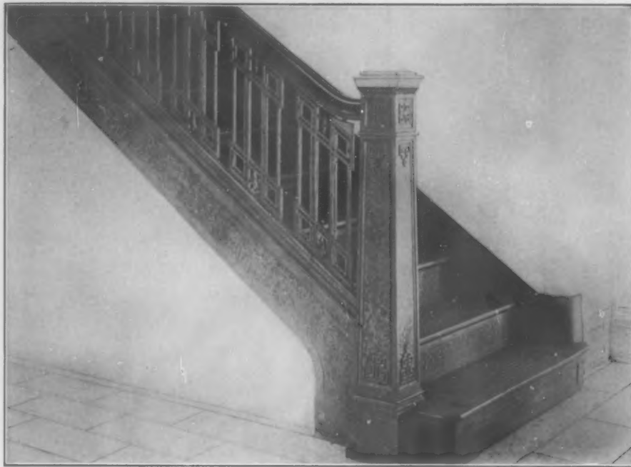
STAIRWAY, R. A. LONG OFFICE BUILDING, KANSAS CITY, MO. Howe, Hoy & Cutler, Architects
