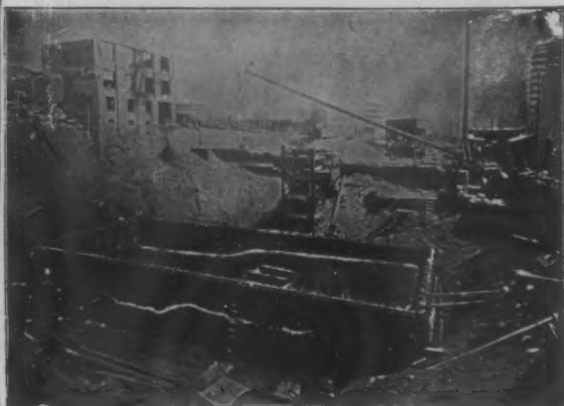
Picture of water-proofed concrete swimming pool. Olympic Club Bldg., San Francisco, California. Thompson-Starrett Co., General Contractors. WRITE FOR PAMPHLET.
