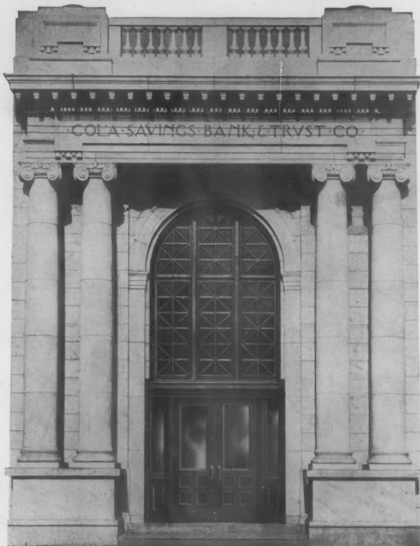
OLD COPPER ENTRANCE COLUMBIA SAVINGS BANK Shand and La Pave, Architects, Columbia, S. C.
