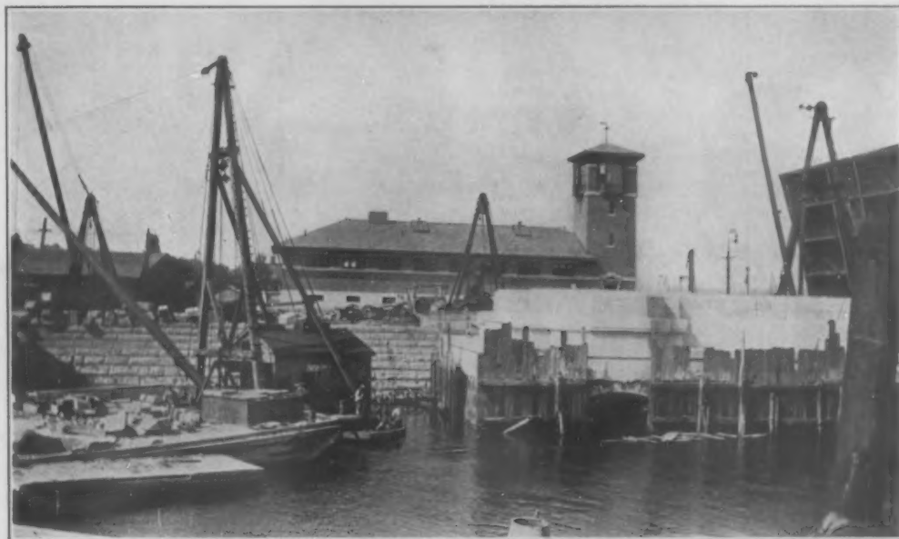
LOWER LOCK GATE HOUSE
