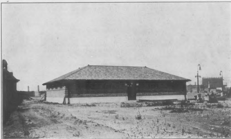
UPPER LOCK GATE HOUSE
