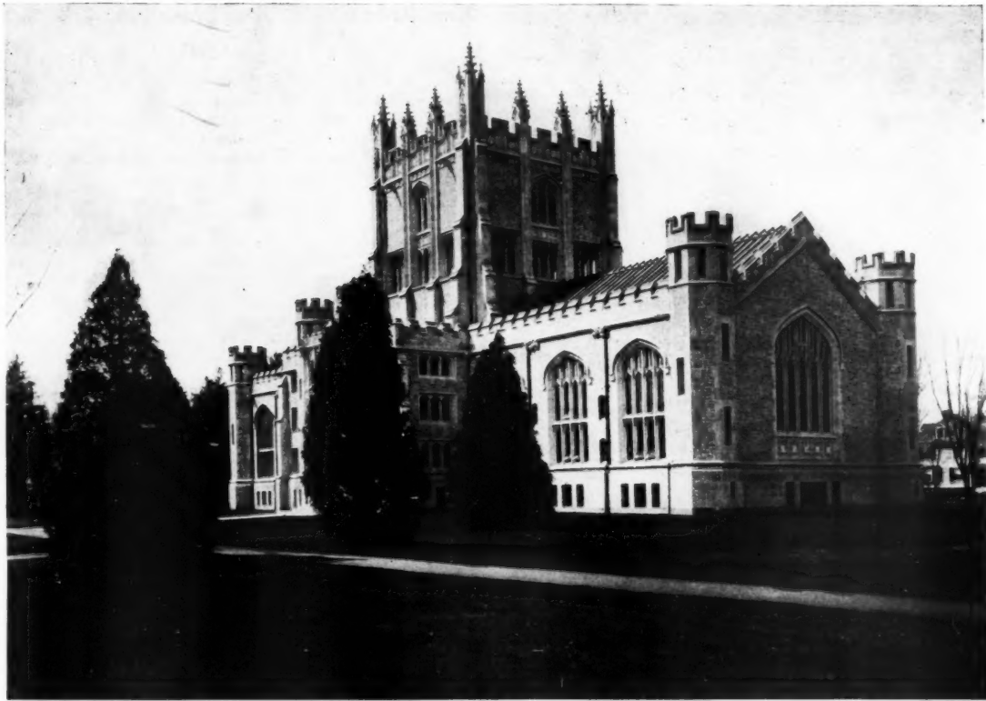
Allen & Collens Architects Boston
