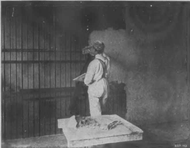
Plastering Lath Surface of HY-RIB
