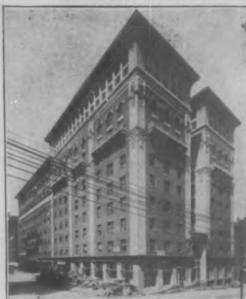
Baltimore Hotel, Kansas City, Mo. Architect, Louis Curtis Berger "Prong Lock" Steel Studs installed.
