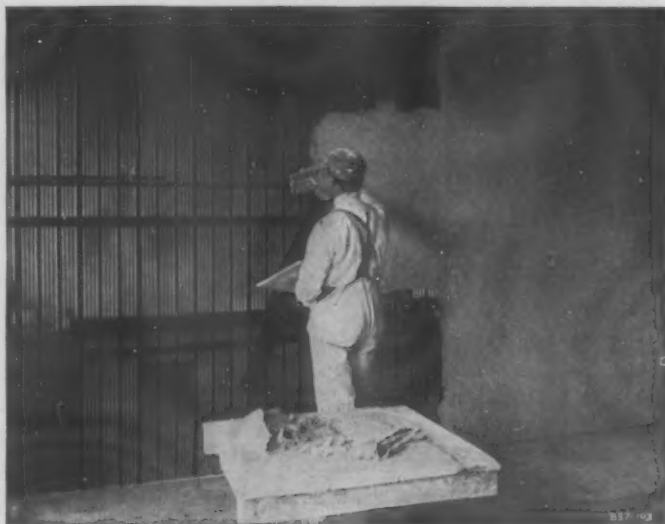
Plastering Lath Surface of HY-RIB
