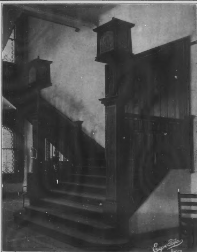
Stairway Wagoner Undertaking Co. Bldg., St. Louis, Mo. F. C. Bonsack Architect
