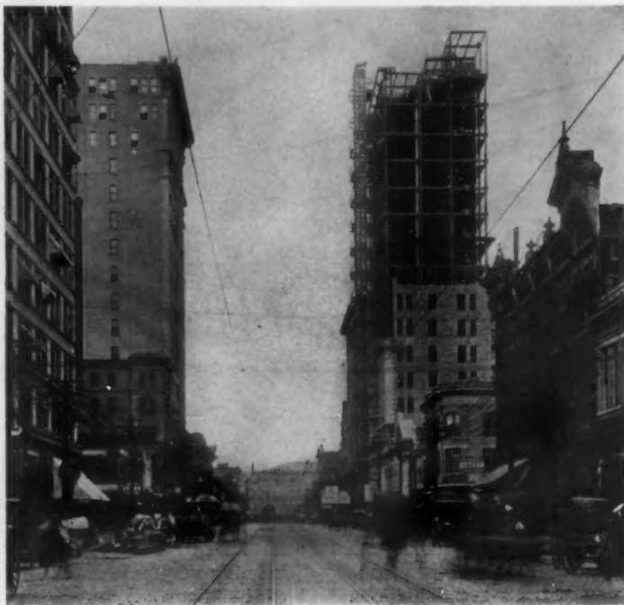
THE BROWN-MARX BUILDING
