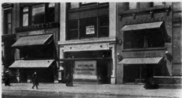
TWO SHOPS SHOWING THE SOMEWHAT UNSATISFACTORY USE OF AWNINGS. THE MIDDLE EXAMPLE IS A WHOLE NEW BUILDING FIFTH AVENUE SHOP FRONTS
