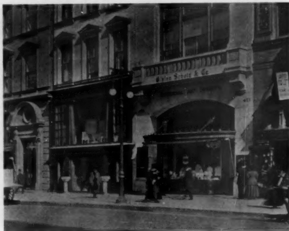
A SHOP FRONT WITH TWO STORIES OF DISPLAY WINDOWS, AND ONE SHOWING AN EFFECTIVE ARCH MOTIVE FOR THE SUPPORT OF THE STORIES ABOVE
