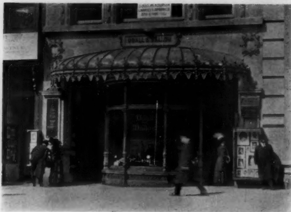
AN INTERESTING VARIATION, WHERE THE WINDOW IS BROUGHT PROMINENTLY FORWARD AND THE ENTRANCES RECESSED
