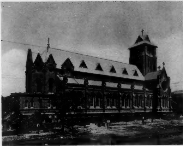
ST. PATRICK'S CHURCH, GALVESTON, TEX. RAISED FIVE FEET UNDER THE DIRECTION OF MR. HARNLEY SHEELER, ENGINEER
