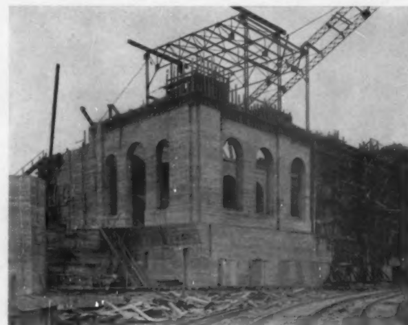
A CORNER OF THE POWER-HOUSE ON THE DOWN-STREAM SIDE, SHOWING THE LOWER TIER OF ARCHES COMPLETED
