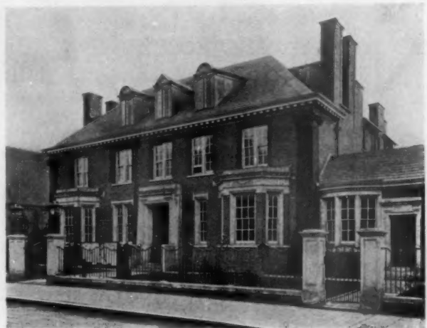
POLICE-OFFICE BUILDINGS SUTTON, SURREY
