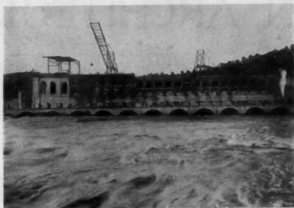
THE POWER-HOUSE FROM BELOW
