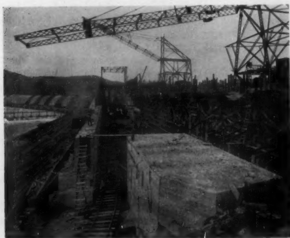
LOOKING ACROSS THE WORK, WITH THE PARTIALLY COMPLETED DAM IN THE DISTANCE
