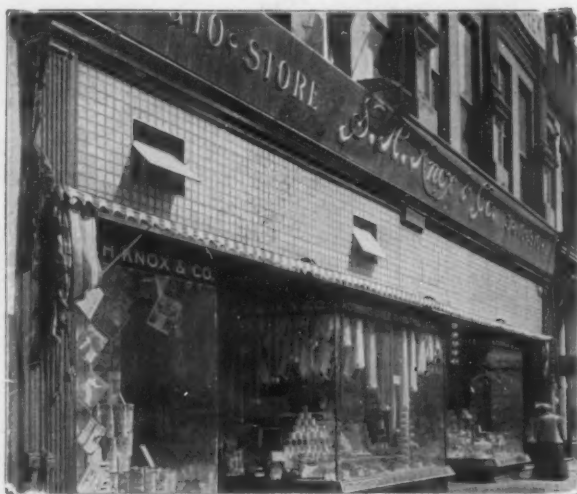
Solid Luxfer transom front with pivoted ventilators.
