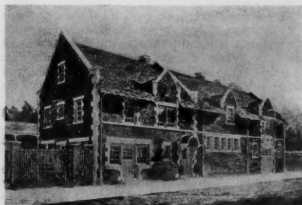
STABLE, OFFICE AND APARTMENT NEWARK WATER DEPARTMENT
