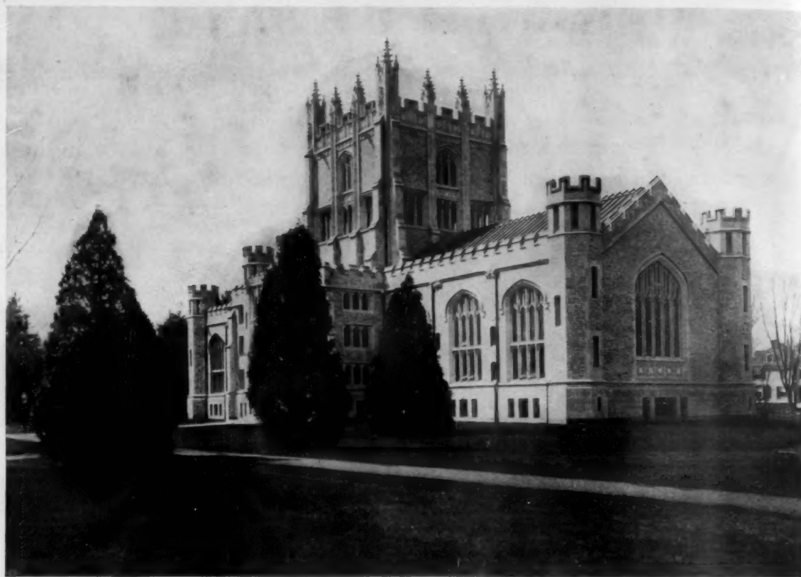
Allen & Collens Architects Boston
