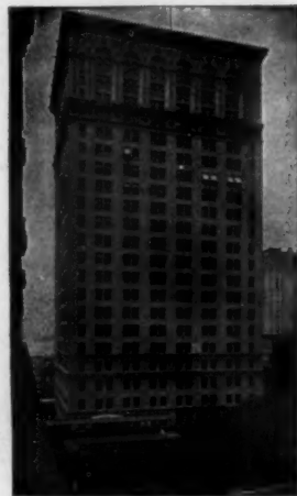
U. S. Express Building, New York. Clinton & Russell, Architects
