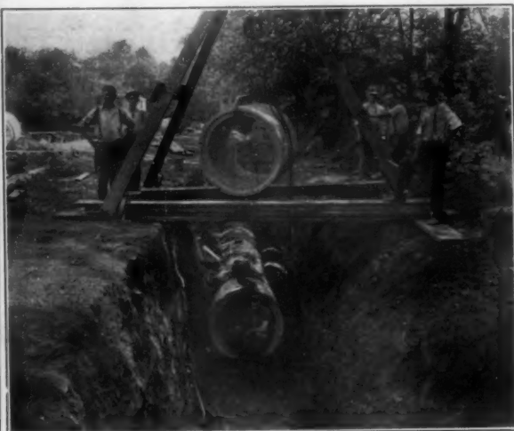
CONCRETE SEWER. WILMINGTON, DEL.
