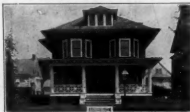
Residence at Forest Hill, N. J. (Sheathed with Neponset), P. T. MacLagan, Architect.
