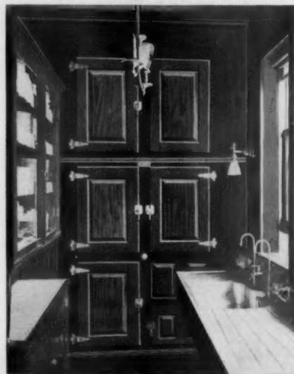
Built to order McCray Refrigerator in the home of Mrs. James H. Barnard, Chicago, Ill. W. Corbys Zimmerman, Architect. Opal glass lining, genuine mahogany exterior to match woodwork of the pantry.
