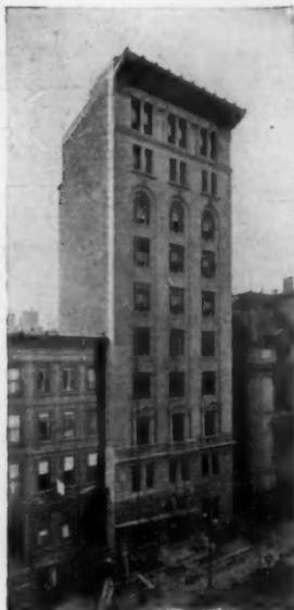
APARTMENT HOUSE, 776 MADISON AV., N.Y. Gordon, Tracy & Swarthout, Architects
