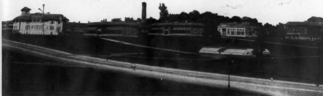
Soldier's Home, Johnson City, Tenn. Covered with "Meurer's Genuine Tinned Iron Sheets."
