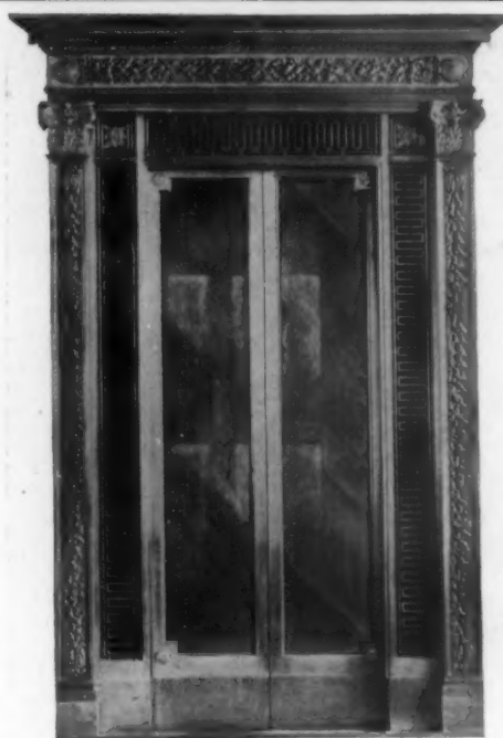
BRONZE ELEVATOR ENCLOSURES, FIRST FLOOR MASSACHUSETTS MUTUAL LIFE INS. CO.'S BUILDING SPRINGFIELD, MASS. TROWBRIDGE & LIVINGSTON, Archts.
