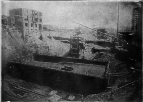
Picture of water-proofed concrete swimming pool. Olympic Club Bldg., San Francisco, California. Thompson-Starrett Co., General Contractors
