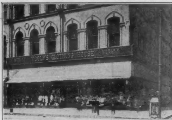
This shows regular transom prism installation above show windows. Note awning attachment.
