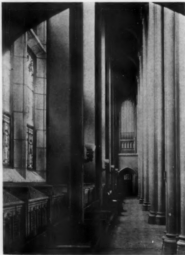
THE AISLE FROM THE REAR OF THE HALL.
