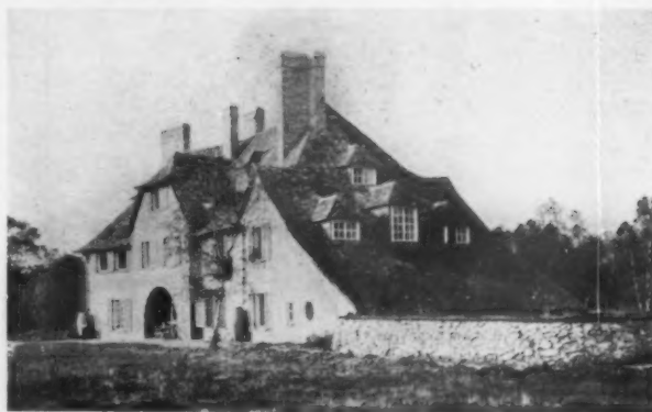
HOUSE AT CHALFONT ST. GILES, BUCKS
