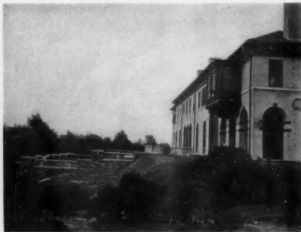
VIEW ALONG TERRACE FRONT
