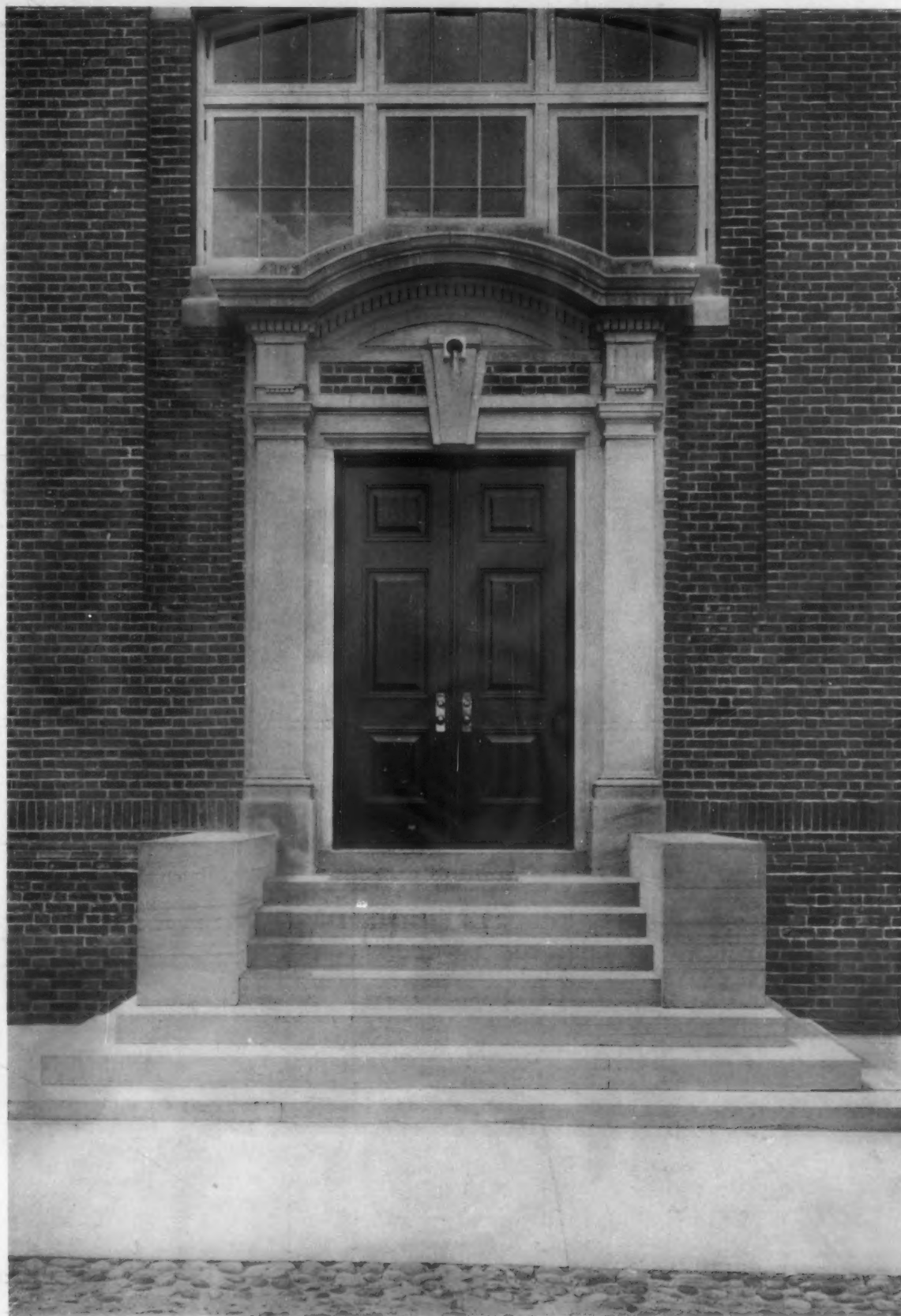
DETAIL OF ENTRANCE
