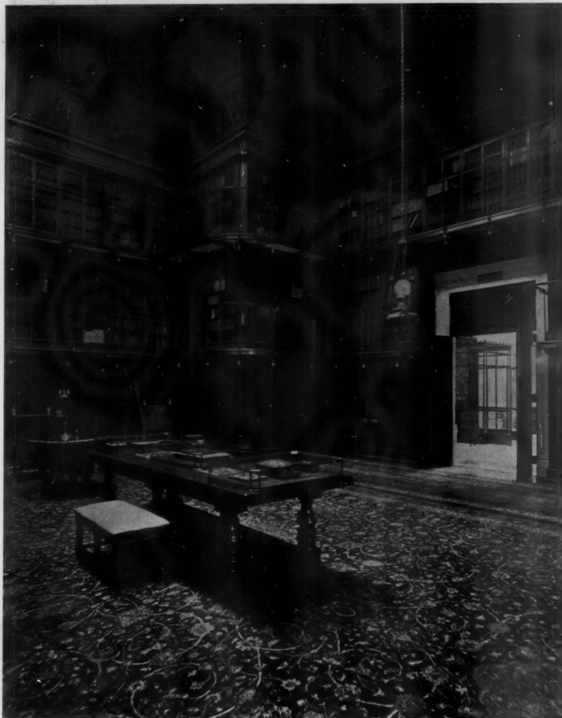
VIEW IN EAST ROOM.
