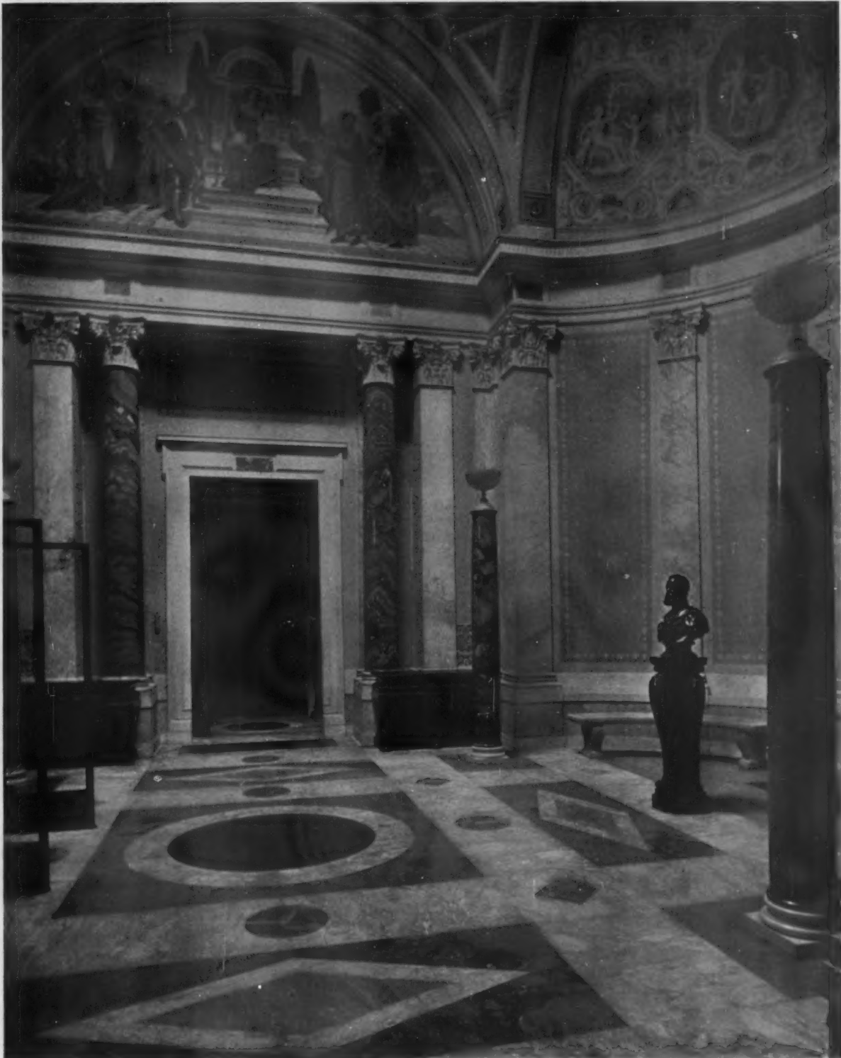
ENTRANCE LOGGIA, LOOKING WEST
