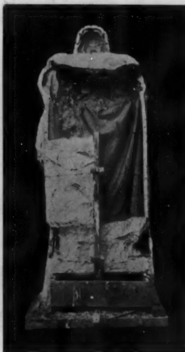
REMOVING CLAY FROM MOULD
