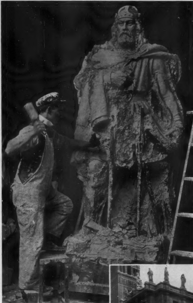
CHIPPING PLASTER MOULD AWAY FROM CAST
