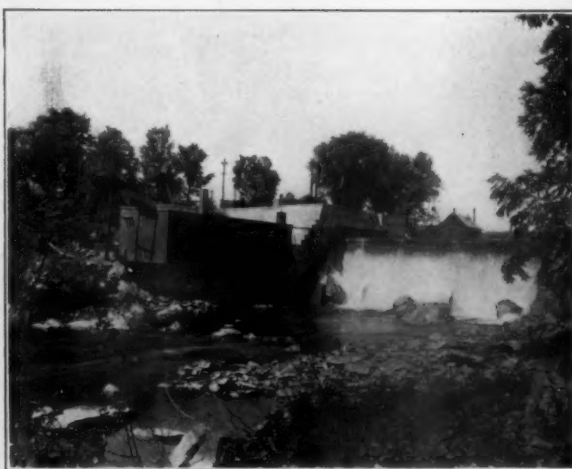
Gravel Concrete Dam, 100 feet long, 36 feet high, built by E. E. Davis, Civil Engineer, Northampton, Mass., for Jones & Lamson Power Co., Perkinsville, Vermont.
