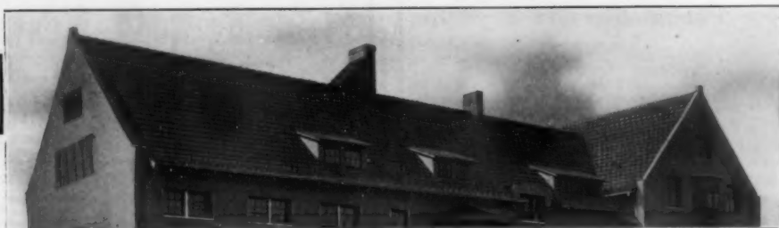
Asbestos "Century" Shingle Roof—Private Stable, Pabst Farms, Oconomowoc, Wis.; Fernekes & Cramer, Milwaukee, Architects; Constructive Sheet Metal Works, Milwaukee, Roofing Contractors
