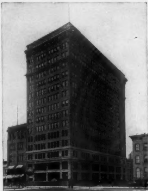
New building of the International Harvester Co. in Chicago. Equipped with
