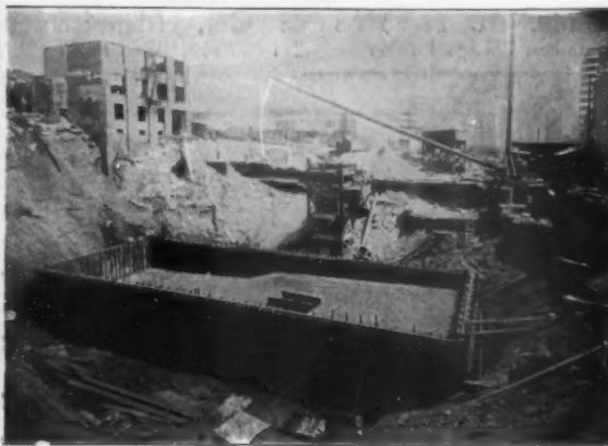
Picture of water-proofed concrete swimming pool. Olympic Club Bldg., San Francisco, California. Thompson-Starrett Co., General Contractors
