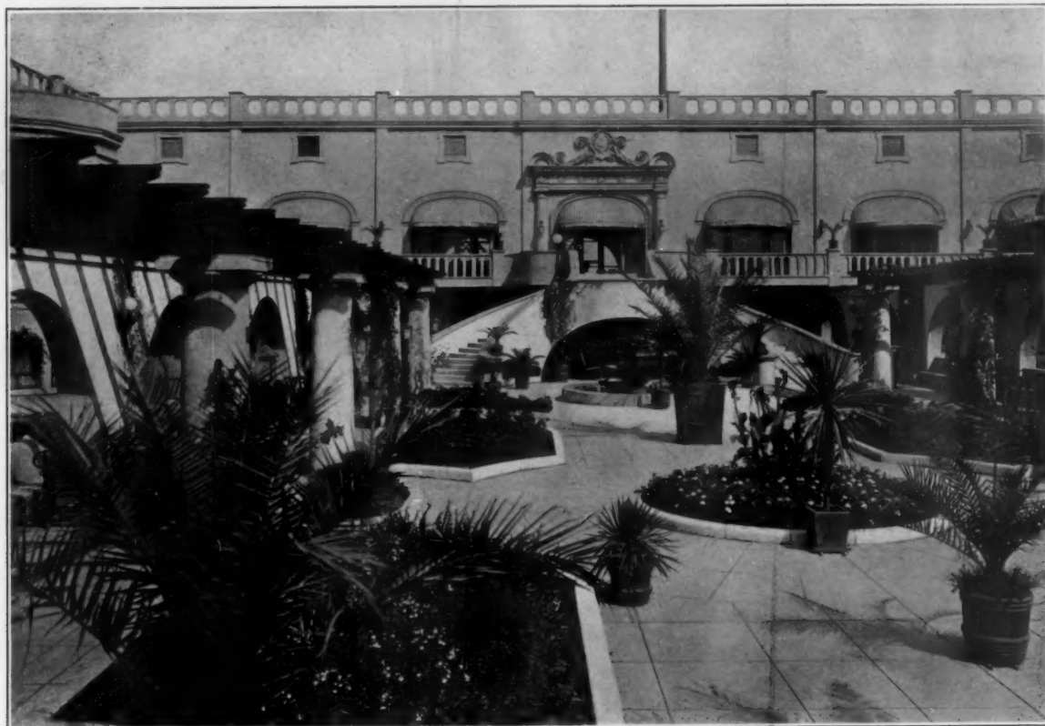
ROOF GARDEN, LOOKING NORTH
