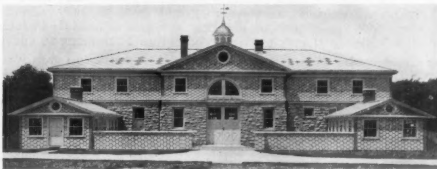
Asbestos "Century" Shingle Roof and Sheathing—Bushy Park, Newport, R. I. J. D. Johnson, Newport, Architect; B. F. Tanner, Newport, Builder
