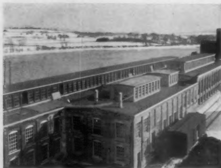
Completed Ferroinclave Roof
