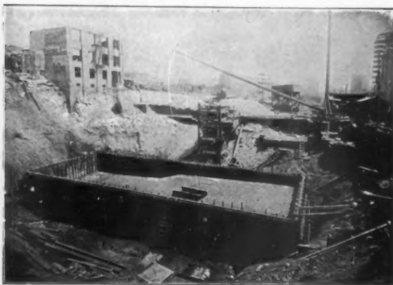
Picture of water-proofed concrete swimming pool. Olympic Club Bldg., San Francisco, California. Thompson-Starrett Co., General Contractors WRITE FOR PAMPHLET
