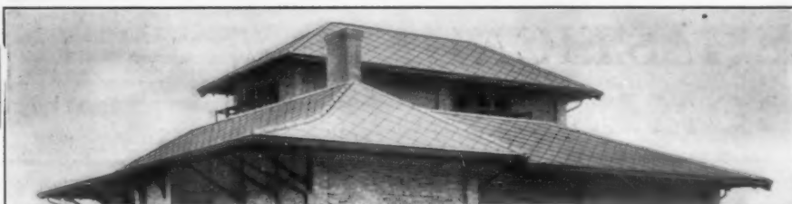
Asbestos "Century" Shingle Roof—Cedarburg Station, Milwaukee Northern Railway Company Comstock Haigh-Walker Company, Contractors
