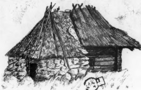
BUILDING ON A FARM AT PÜHHALEP, ESTHONIA on the Baltic, showing combination of kitchen and bath houses under one thatch. Bathhouse of stone, kitchen of timber.
