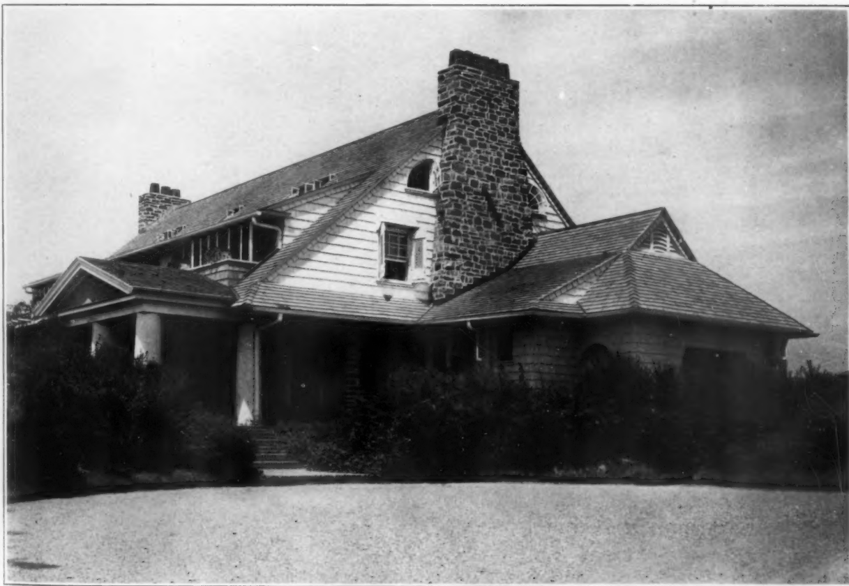
DETAILS, HOUSE NO. 1, WOODMERE, L. I., N. Y. MR. CHARLES BARTON KEEN, ARCHITECT.
