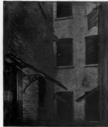
Showing arrangement of Prism Canopies over Windows
