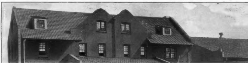
Asbestos "Century" Shingle Roof.—Clubhouse and Office, Pabst Farms, Oconomowoc Wis Fernekes & Cramer. Architects Milwaukee; Consolidated Sheet Metal Works, Roofing Contractors, Milwaukee
