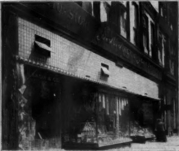
Solid Luxfer transom front with pivoted ventilators.
