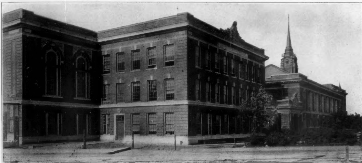
VIEW LOOKING NORTH FROM HUNTINGTON AVENUE.
