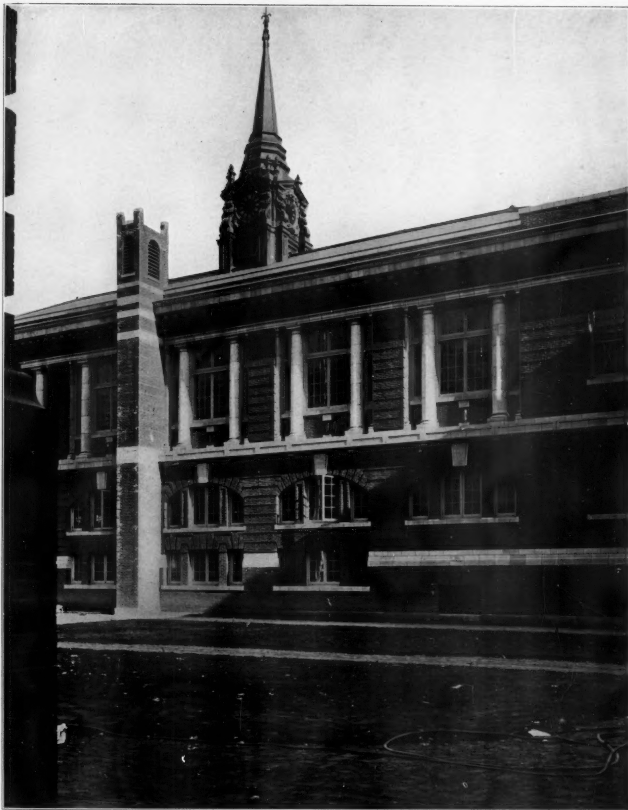
DETAIL OF COURTYARD, FRONT OF COMMON BUILDING.
