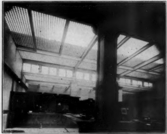
Berger Raydiant Lights in accounting room below court, First National Bank, Birmingham, Ala.
