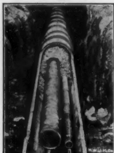
J-M Conduit After Ten Years' Service
