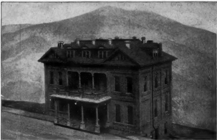
Hospital erected by the United Verde Copper Co., Jerome, Ariz., using 2 24-inch and 7 18-inch "Burt" glass top ventilators. Other hospitals using "Burt" Ventilators are: Mercy Hospital, Pittsburg; State Sanatorium for Treatment of Tuberculosis, Howell, Mich.; St. Luke's Hospital, Utica, N. Y.; Akron City Hospital, Akron, Ohio.
