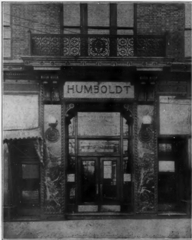
BRONZE ENTRANCE HUMBOLDT BUILDING, ST. LOUIS Mauran Russell & Garden, Architects.
