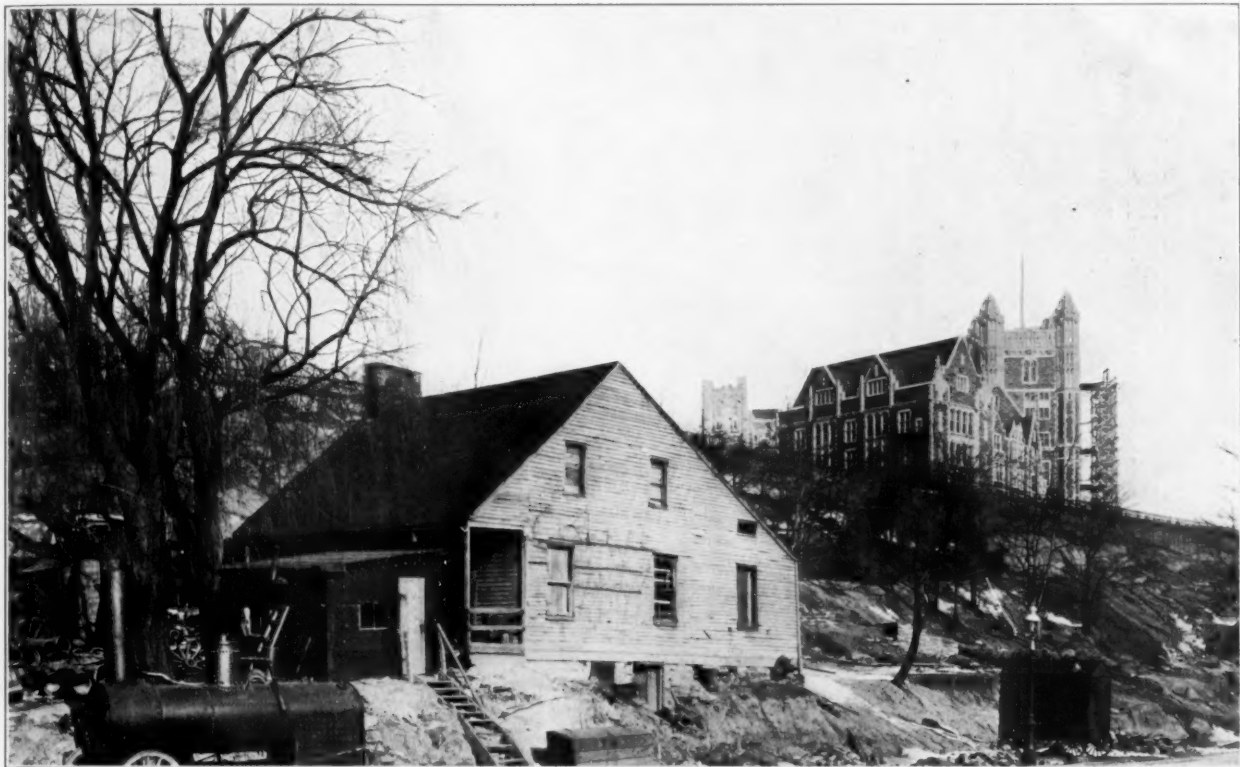
VIEW OF MAIN BUILDING FROM SOUTHEAST.
