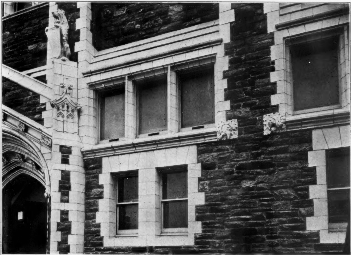
GYMNASIUM BUILDING DETAIL.
