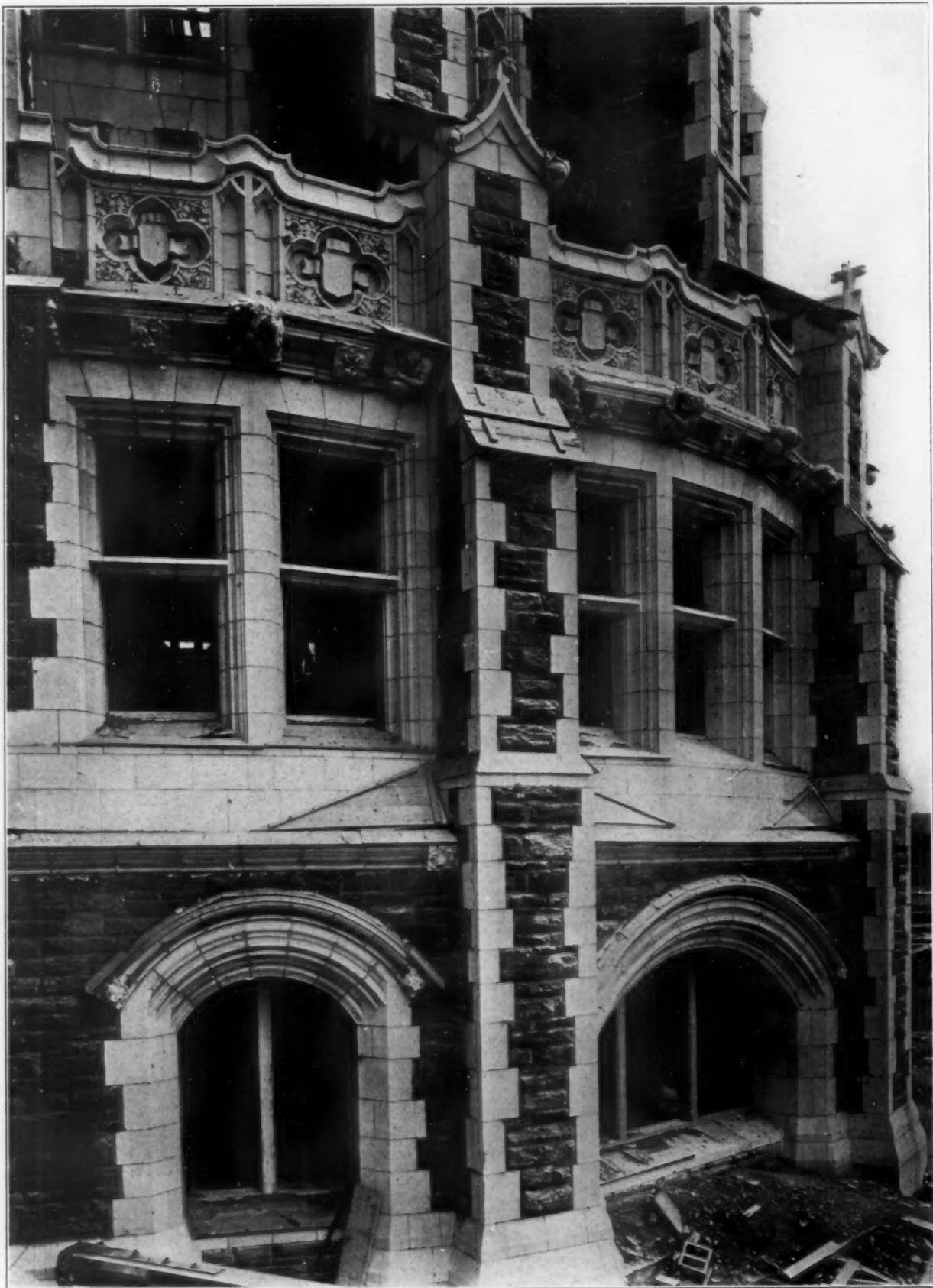
DETAIL OF LIBRARY—MAIN BUILDING. COLLEGE OF THE CITY OF NEW YORK.
