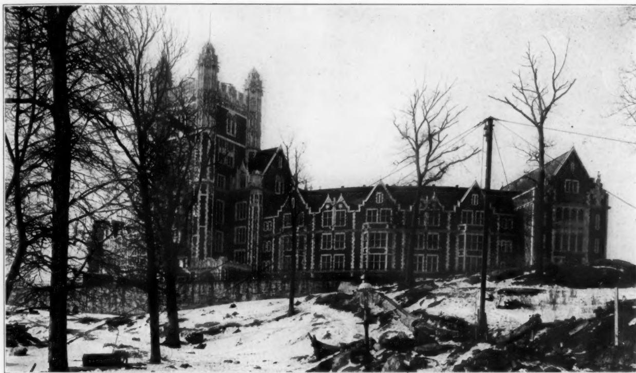
MAIN BUILDING FROM THE NORTH.
