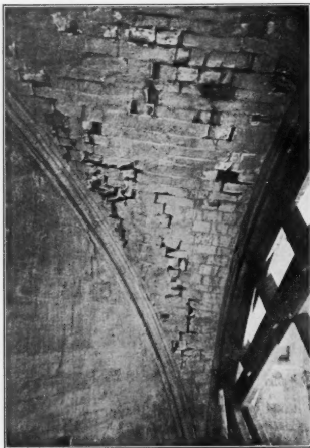
FIG. 5.—WINCHESTER CATHEDRAL. DISINTEGRATED CONDITION OF VAULTING AT PRESBYTERY.
