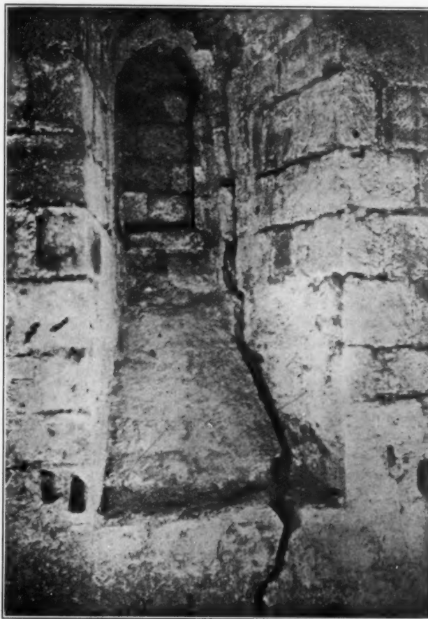
FIG. 6.—WINCHESTER CATHEDRAL. CRACK IN WINDOW, MAIN CRYPT.
