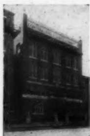
Branch Carnegie Library, Architects, Messrs. Babb, Cook & Willard, New York. Built on Raymond Concrete Piles.
