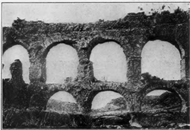
ARCHA DELLA MOLA, AN ANCIENT ROMAN AQUEDUCT.
