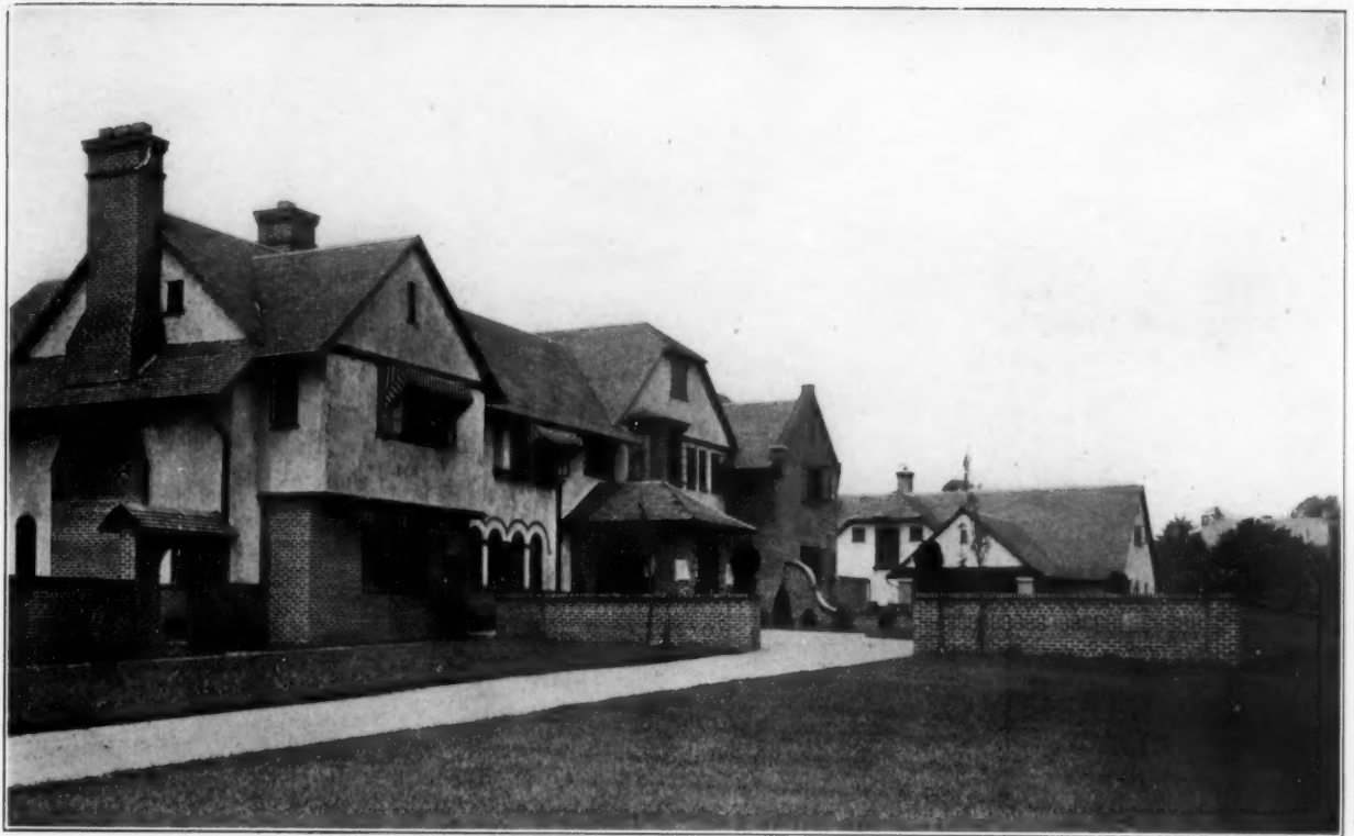
ENTRANCE FRONT: HOUSE OF MR. MAXWELL WYETH, ROSEMOUNT, PA.
