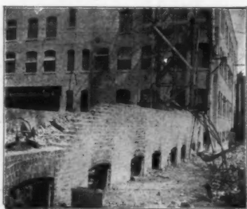
REAR VIEW NEW BUILDING, SHOWING GENERAL CONDITION OF VOIGTMANN WINDOWS AFTER FIRE Myerford Factory, Chicago, Ill., engulfed in flames for three hours without loss to building or contents
