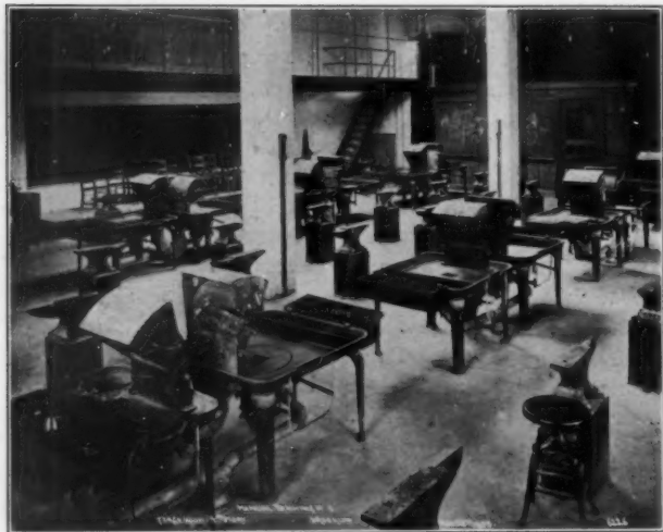
FIG. 2. FORGE ROOM: MANUAL TRAINING HIGH SCHOOL.
