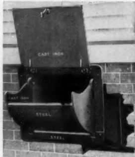
Showing door locked open protecting the siding
