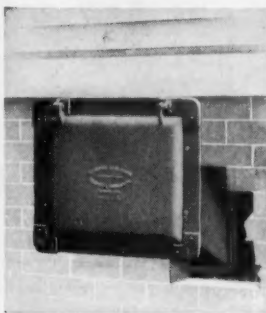
Showing door closed and automatically locked
