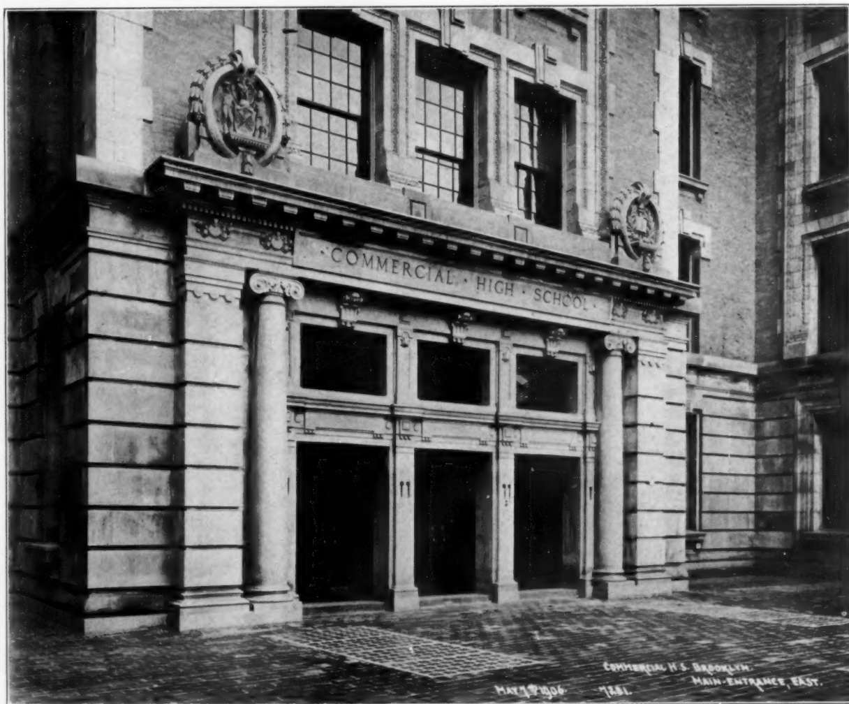
PLATE 42. ENTRANCE DETAIL: COMMERCIAL HIGH SCHOOL, BROOKLYN.
