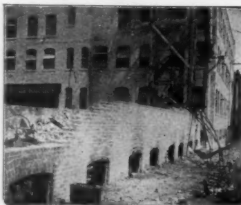
REAR VIEW NEW BUILDING, SHOWING GENERAL CONDITION OF VOIGTMANN WINDOWS AFTER FIRE
