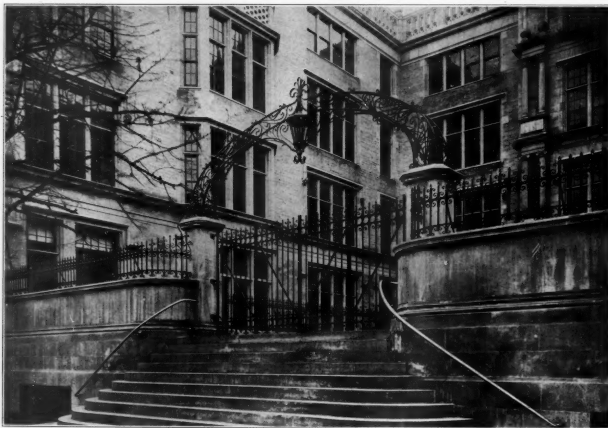
PLATE 32. PUBLIC SCHOOL NO. 37, BRONX: SOUTH GATE. PUBLIC SCHOOL BUILDINGS, NEW YORK, N. Y. C. B. J. Snyder, Architect.
