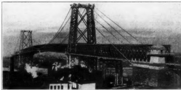
THE WILLIAMSBURG BRIDGE, NEW YORK.
