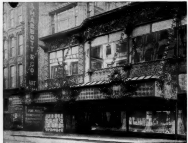
How Luxfer 4-in. squares combine in securing highly ornamental structural effects.
