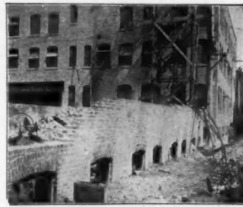
REAR VIEW NEW BUILDING, SHOWING GENERAL CONDITION OF VOIGTMANN WINDOWS AFTER FIRE Myercord Factory, Chicago, Ill., engulfed in flames for three hours without loss to building or contents
