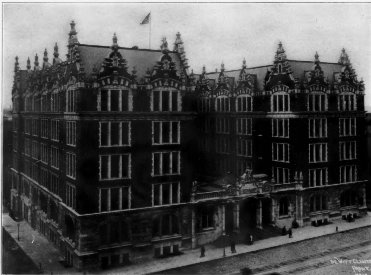
PLATE 18. VIEW FROM SOUTHEAST.
