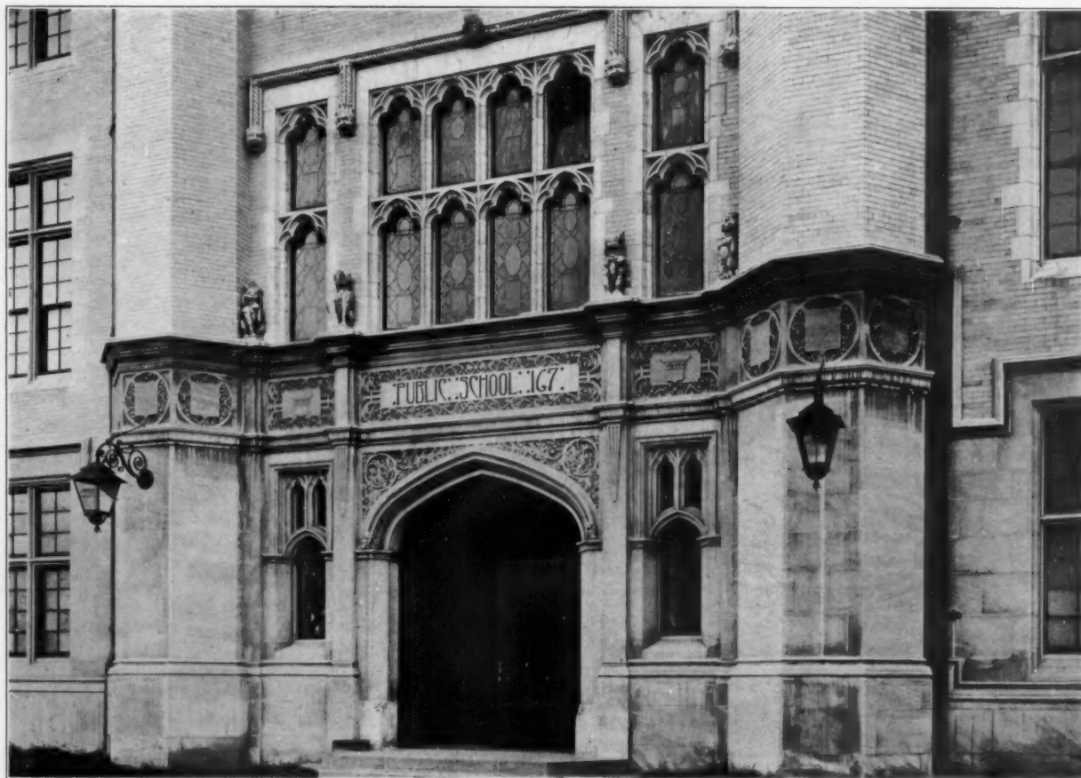
PLATE 23. DETAIL MAIN ENTRANCE.
