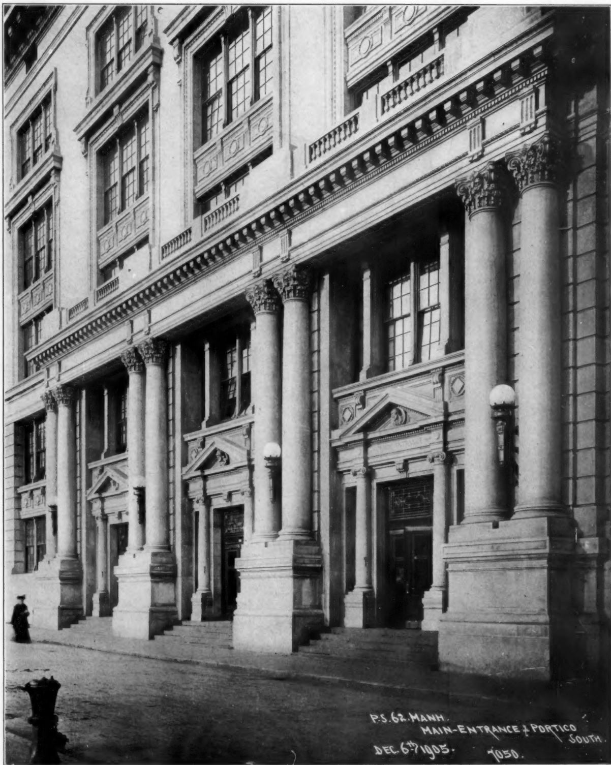
PLATE I. MAIN ENTRANCE AND PORTICO: PUBLIC SCHOOL NO. 62, FLESTER, ESSEX AND NORFOLK STREETS.
