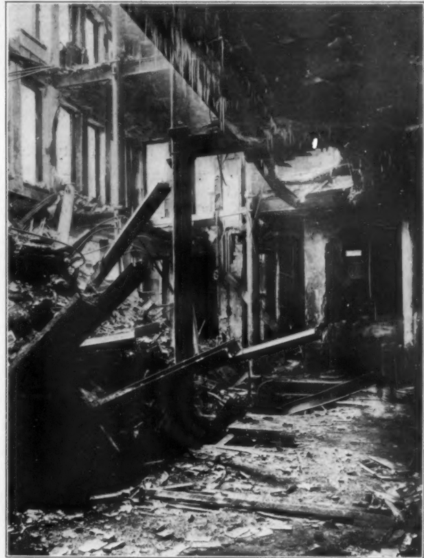
VIEW ON FIRST FLOOR, LOOKING SOUTH.
