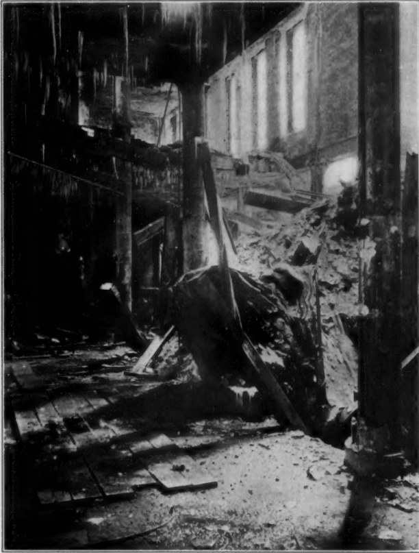
VIEW ON FIRST FLOOR, LOOKING EAST.
