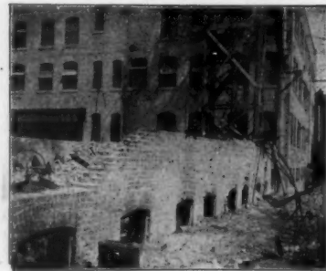
REAR VIEW NEW BUILDING, SHOWING GENERAL CONDITION OF VOIGTMANN WINDOWS AFTER FIRE Myerford Factory, Chicago, Ill., engulfed in flames for three hours without loss to building or contents
