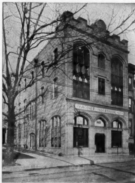
WAGONER UNDERTAKING CO. BUILDING, ST. LOUIS.
