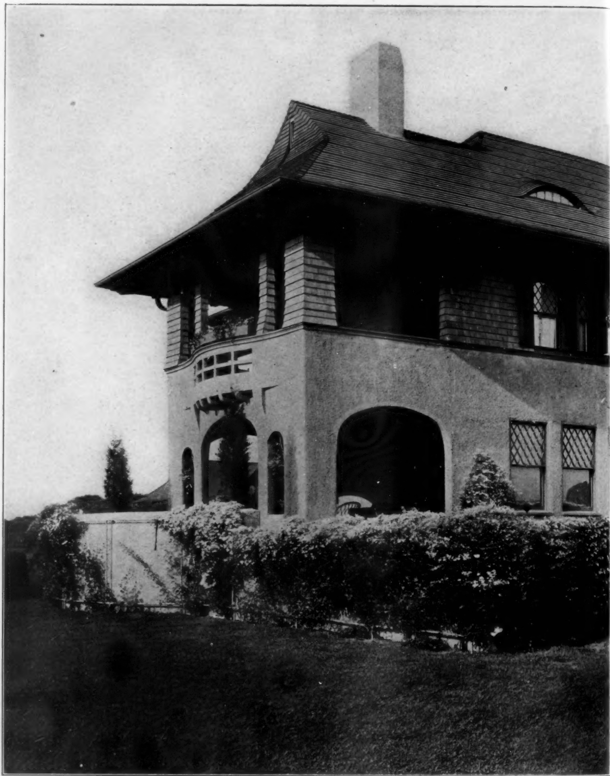
DETAIL OF LOGGIA AND TERRACE: HOUSE OF DR. A. H. ELY, SOUTHAMPTON, LONG ISLAND, N. Y.
