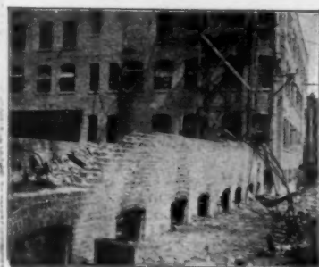
REAR VIEW NEW BUILDING, SHOWING GENERAL CONDITION OF VOIGTMANN WINDOWS AFTER FIRE
