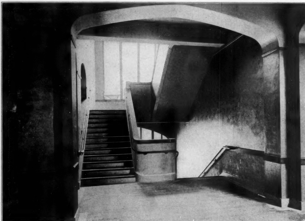
CONCRETE STAIRWAY, LAFAYETTE SCHOOL.
