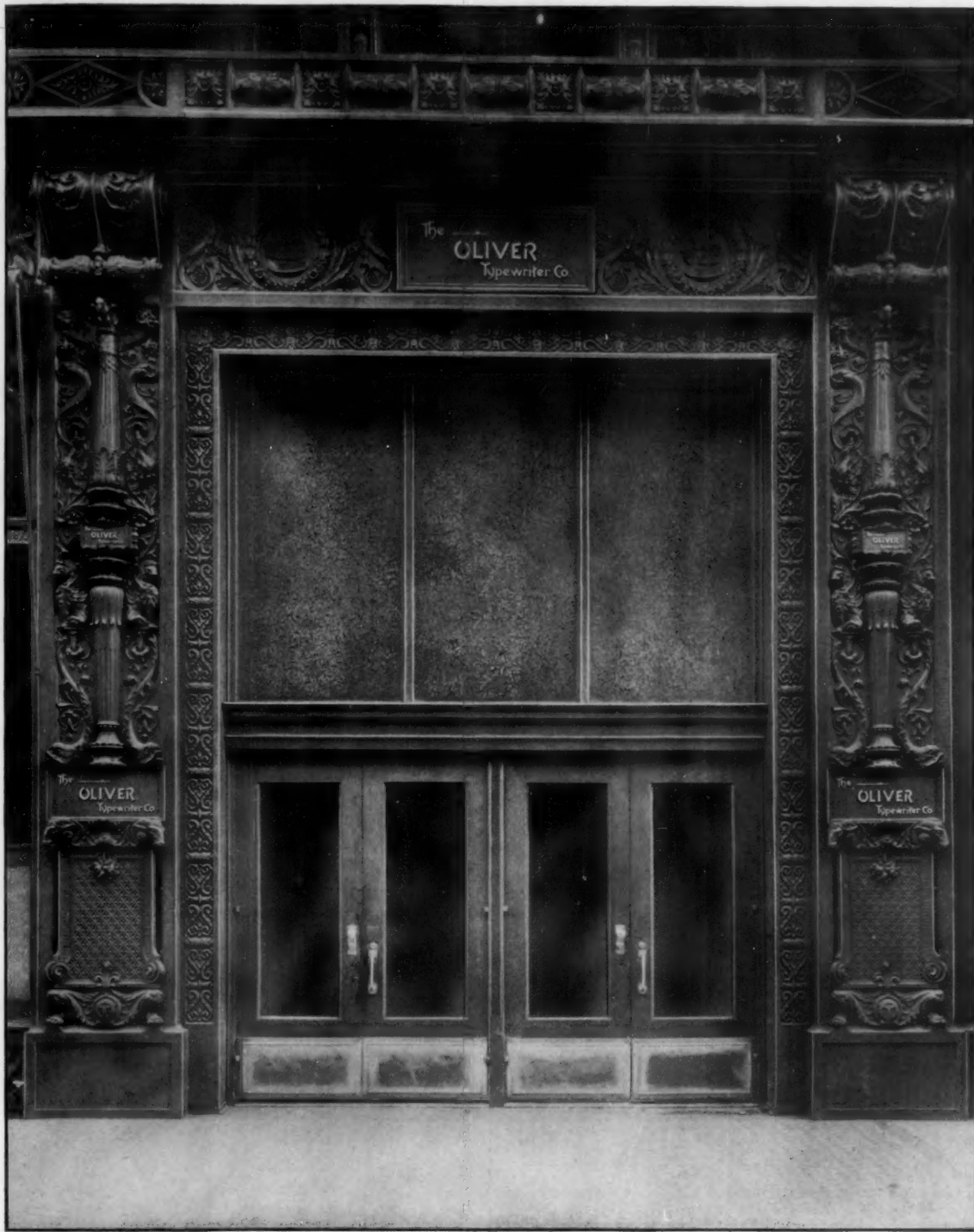
ENTRANCE DETAIL CAST IRON FRONT, OLIVER TYPEWRITER BUILDING, CHICAGO HOLABIRD AND ROCHE, ARCHITECTS
