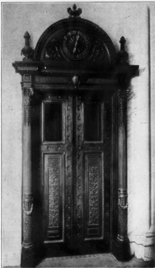
ELEVATOR ENCLOSURE FIRST STORY TRUST CO. OF AMERICA BUILDING, NEW YORK FRANCIS H. KIMBALL, ARCHITECT
