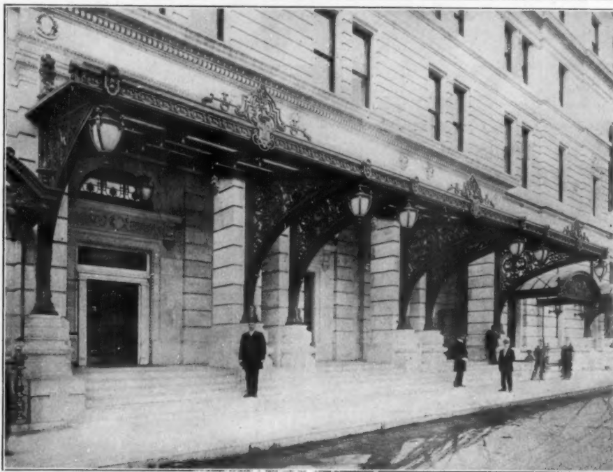
MAIN CANOPY—59th STREET SIDE: PLAZA HOTEL, NEW YORK. H. J. Hardenbergh, Architect.
