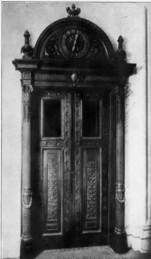
ELEVATOR ENCLOSURE FIRST STORY
