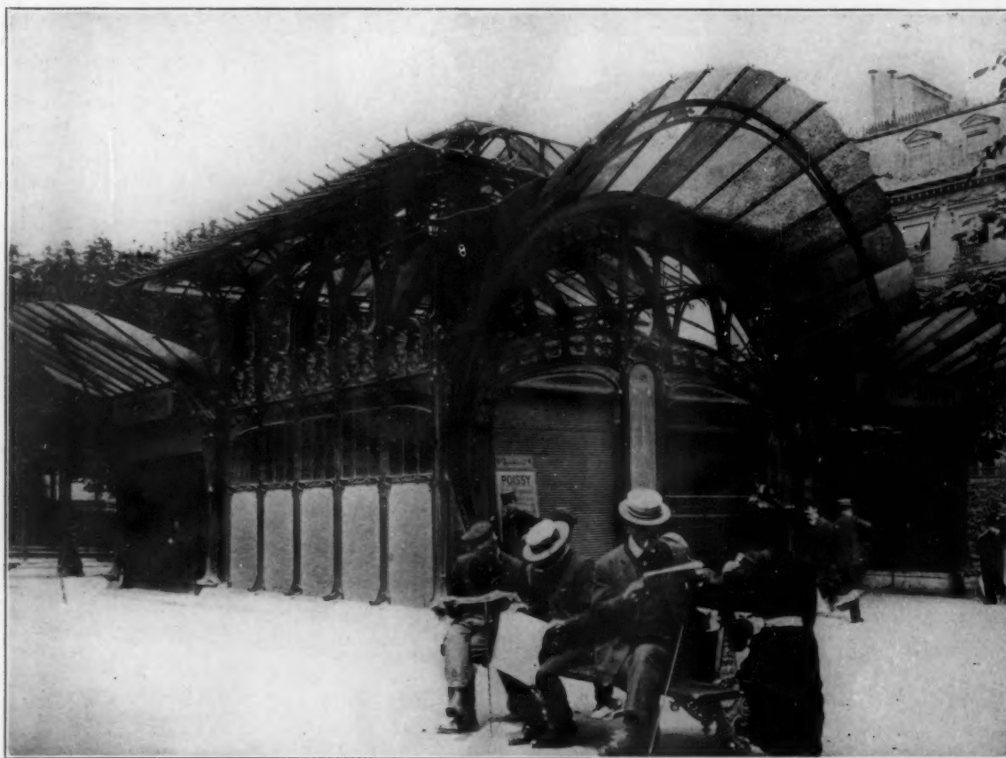
SUBWAY STATION, PLACE DE L'ÉTOILE, PARIS.
